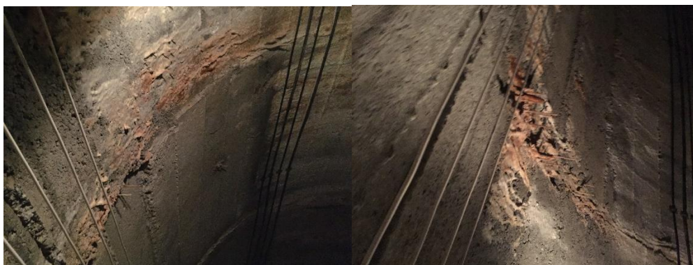
Fig. 3. The emergency sections of underground tunnel
